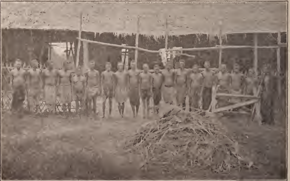
Force of Batetela workmen constructing a new house at Luebo to furnish shelter for the large party of new missionaries arriving there recently. These workmen came from their native homes, three months' march from Luebo, and are skilful house builders.
